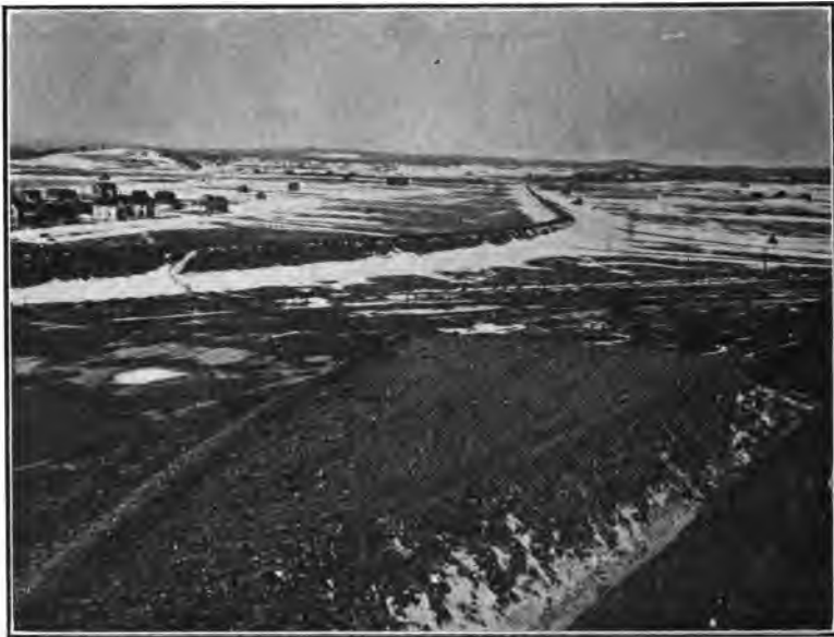
FIGURE 8 CLIFFS SHAFT MINE—LUMP ORE PILE, SHOWING METHOD OF FANNING OUT FROM TRESTLE
